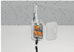
Pendant light connection in a suspended ceiling
