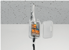
Pendant light connection in a suspended ceiling
